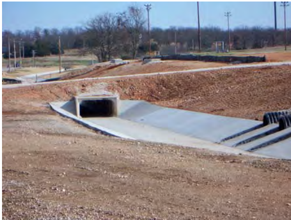
25. Replacement Avenue Noncontributing concrete culvert/bridge and poured concrete ditch
