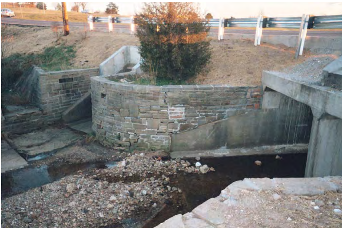
Figure 84. Example of inappropriate mortar replacement and new concrete without tinting at the Nebraska/Minnesota Culvert (ERDC-CERL).
