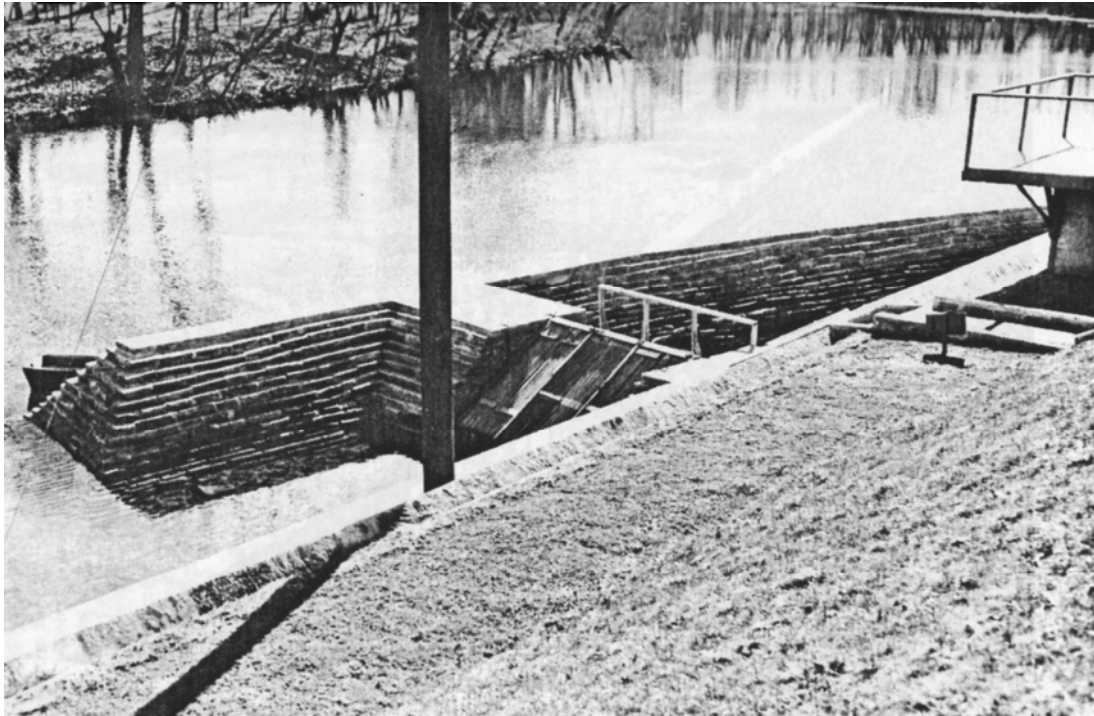
Figure 35: Stone boat landing under construction by POWs at Fort Leonard Wood, 1944 (U.S. Army Signal Corps photo in Bartholomew & Associates, 30).
