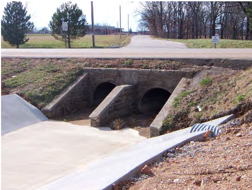
Figure 85. Example of inappropriate new concrete culvert without tinting at the Constitution Avenue Culvert (ERDC-CERL).
