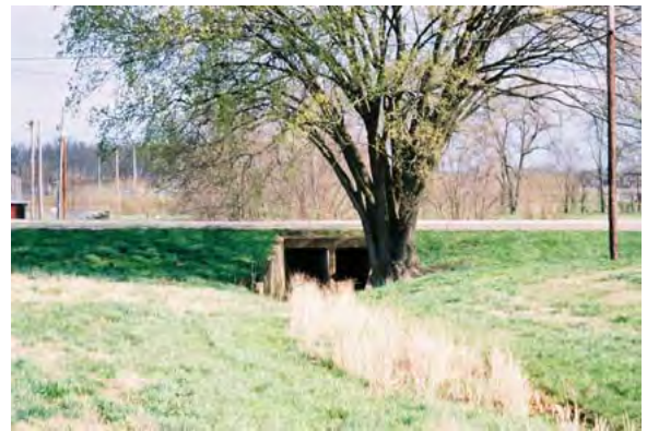
8. Kansas Avenue Noncontributing poured concrete culverts
