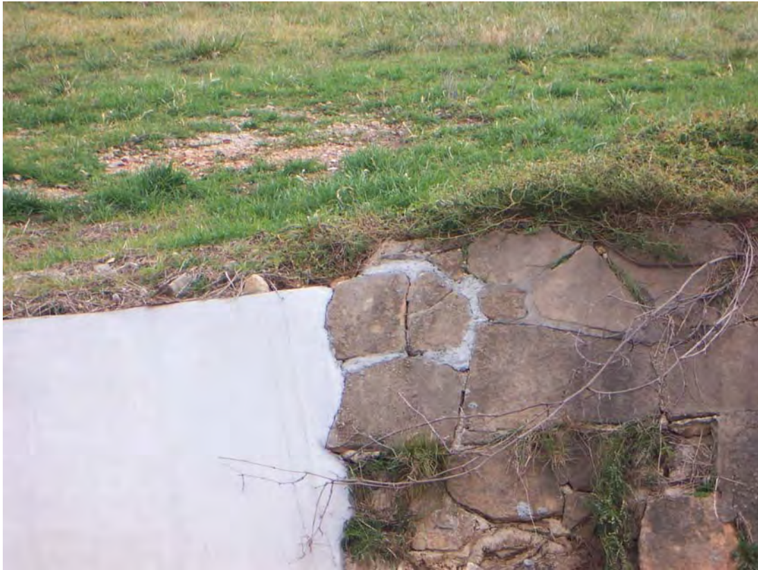
Figure 83. Example of inappropriate mortar replacement and new concrete without tinting at the Nebraska/Minnesota Culvert (ERDC-CERL).
